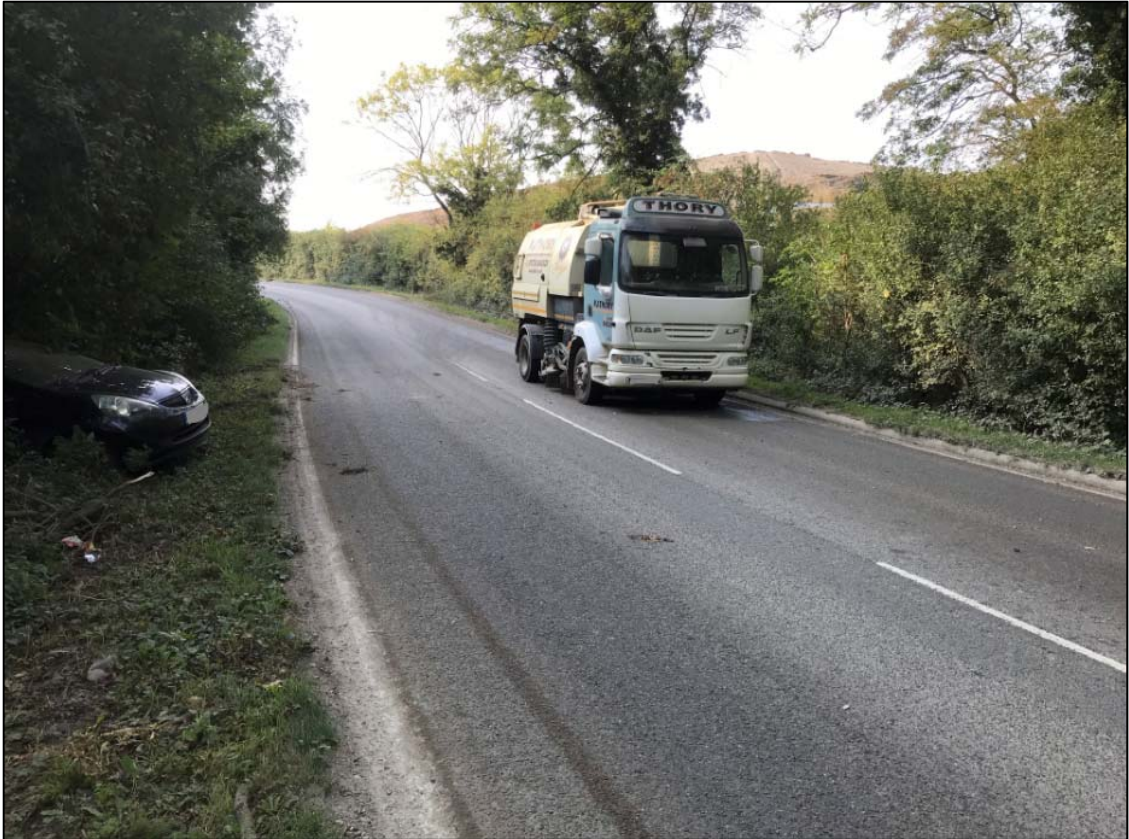
Image 2.2 – Damage Only Accident 17 th September 2020
